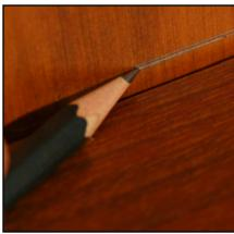
Most laminate installations involve areas covered by the arc of a swinging door, and even though laminates are relatively thin, you'll probably still need to trim the bottom of your doors to accommodate the raised floor.
